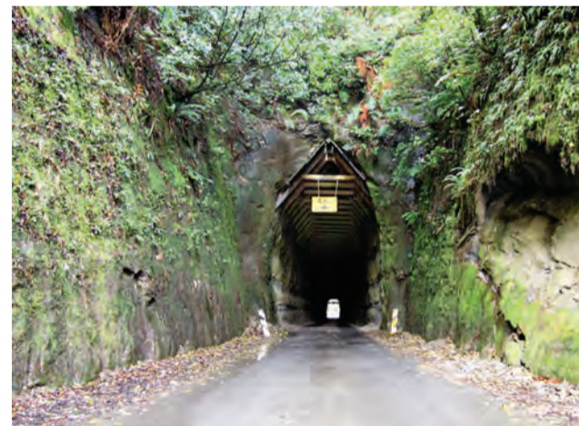
The single lane tunnel on the highway.
